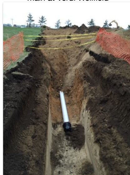
Installation of new raw water main at Verdi Wellfield
