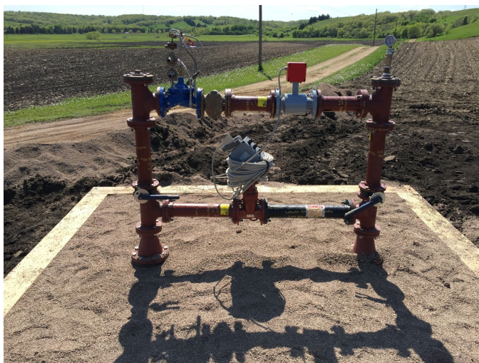
New above ground meter and control structures, City of Lake Benton
